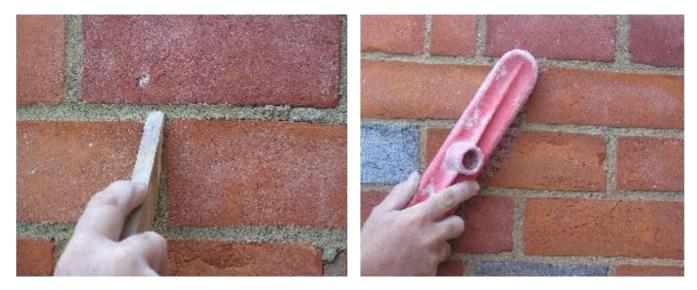
**NOTE:** If mortar gets onto the face of the brickwork/ stonework brush or beat it off when it is dry. Removal whilst the mortar is wet will spread staining. Stains can be removed using a mild brick acid however; the natural weathering process will remove most stains over the winter period.
